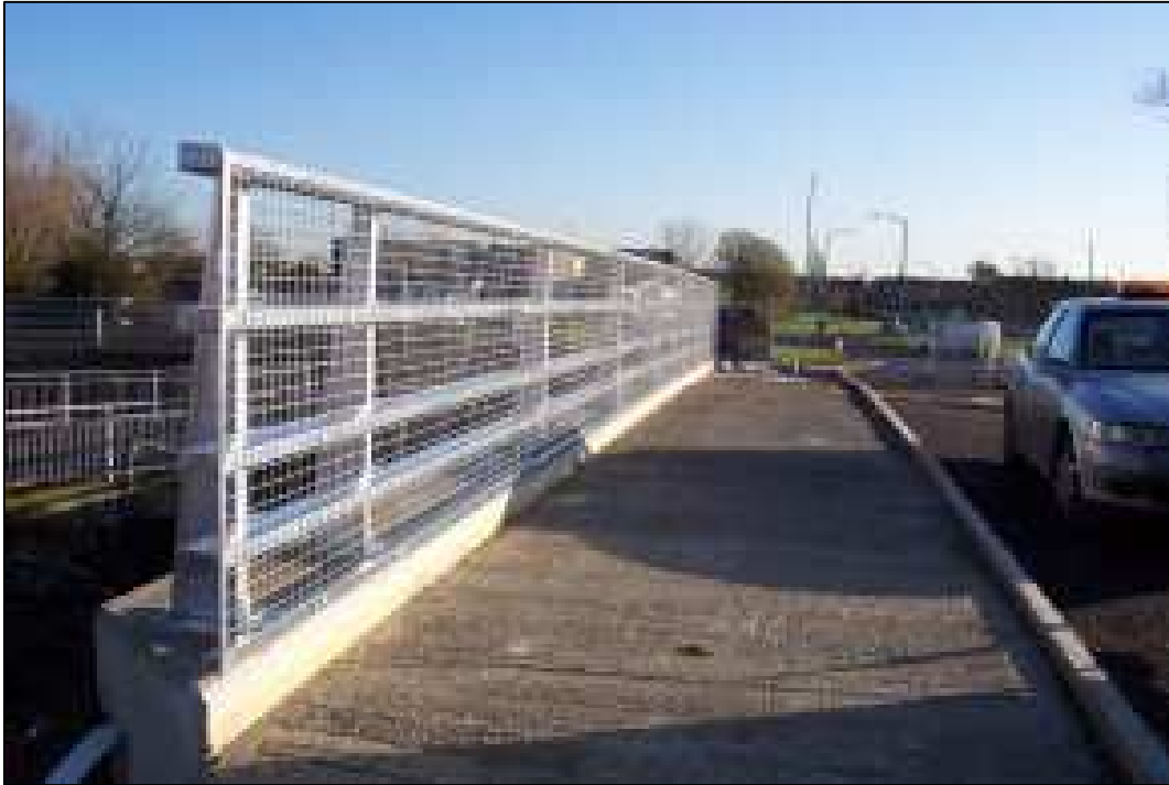
Picture 3: Parapet with mesh
