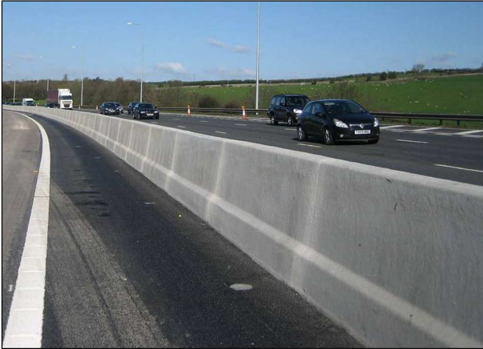
Picture 1: Concrete central reserve barrier
