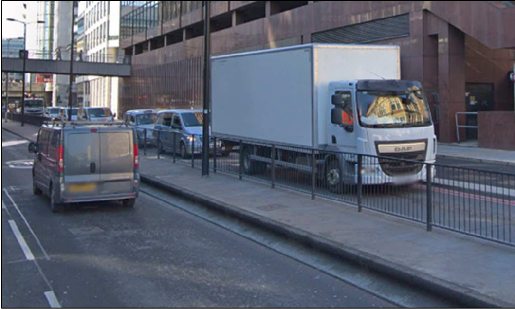
Picture 2: Trief kerb and pedestrian guardrail
